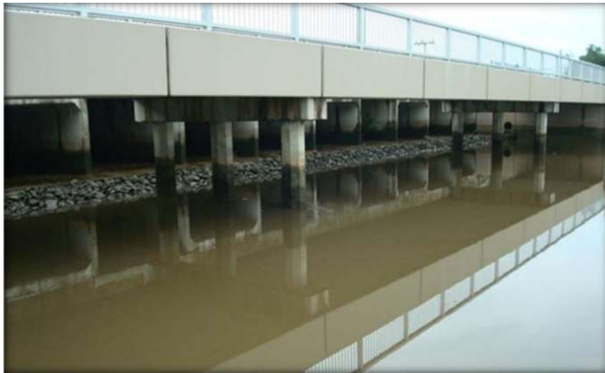
Figure 5. Upstream - Santa Barbara Culverts
